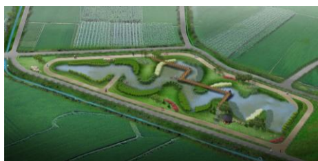
Figure 1. View of constructed stormwater wetland investigated in this study
